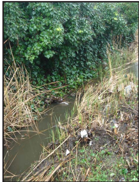
Overgrown in-channel vegetation, due to abandoned maintenance routine, causes flooding
