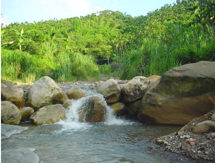
Figure 6.4 A grade control work constructed with Japanese traditional mason techniques
