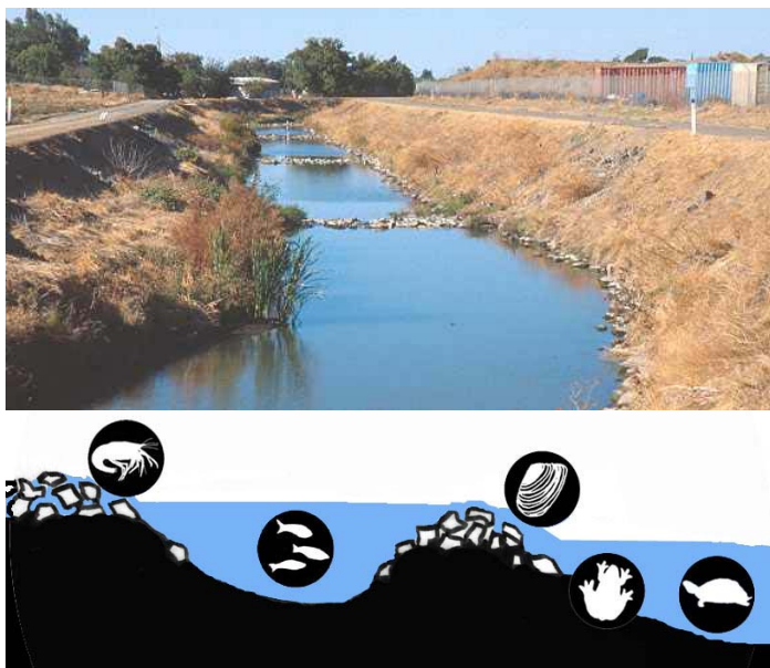
Figure 4.54 The artificial riffles and pools house several species and provide rich wildlife contact. (Up: the stretch of Marsh Creek by Wastewater Treatment Plant. Down: species observed)
