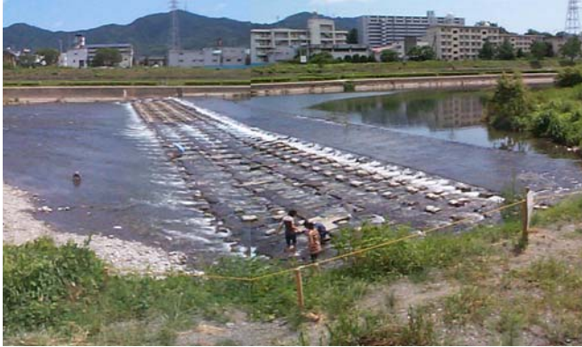
Figure 4.90 The drop work creates erosion at the left bank in Kagami River. Although a poor work from an engineering view point, the area becomes a rich water contact zone
