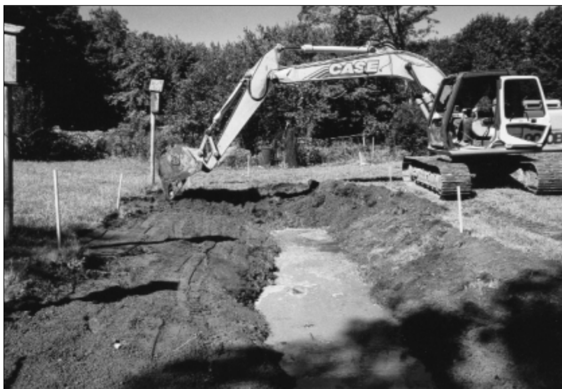
A backhoe halfway through removing a culvert and grading the banks of West Ox Pasture Brook in a Rowley, Massachusetts backyard. Courtesy of Rowley Conservation Commission.
