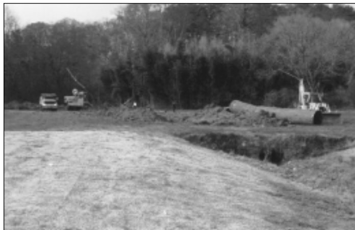
Daylighting is often a good, low-cost solution for collapsed culverts. This 1994 project near Atlanta, Georgia replaced a deteriorating metal pipe with an open, naturalized channel. Courtesy of DeKalb County Parks Department.
