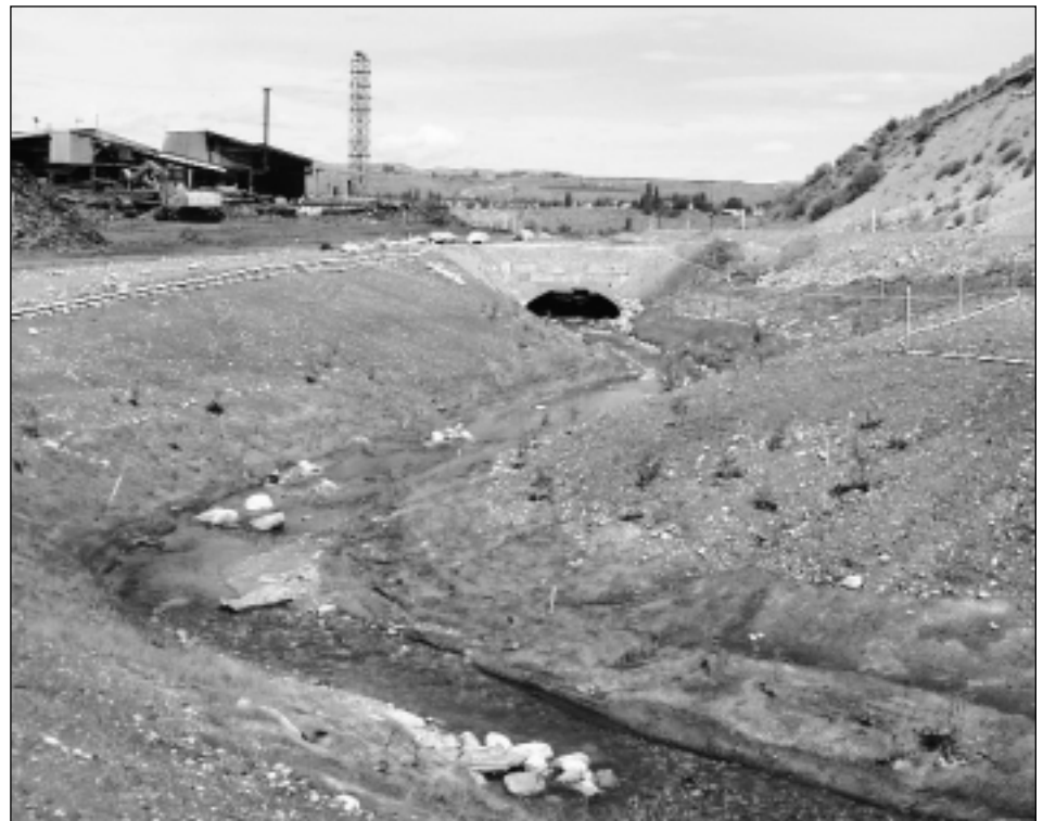
A portion of the daylighting project by the Quality Veneer & Lumber mill in Omak, Washington, a few months after completion in 1999. Vegetation is just beginning to take hold. The new “bottomless culvert” in the upper middle of the photo spans a short stretch of the opened stream. Courtesy of Ridolfi Engineers.
