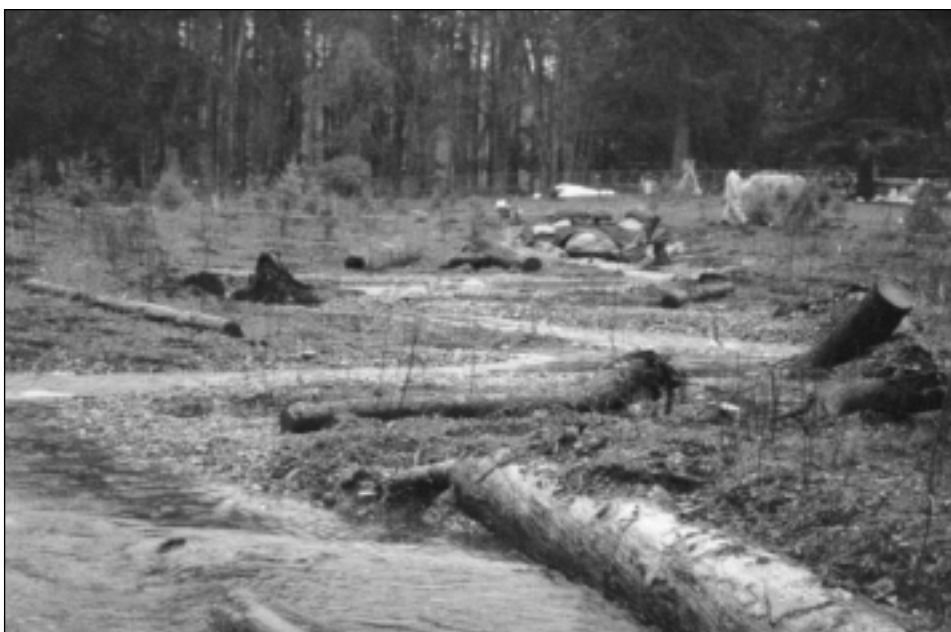
A section of Jenkins Creek shortly after daylighting, showing meanders and newly installed habitat features such as root wads and control logs. Courtesy of Ken Nilsen.
