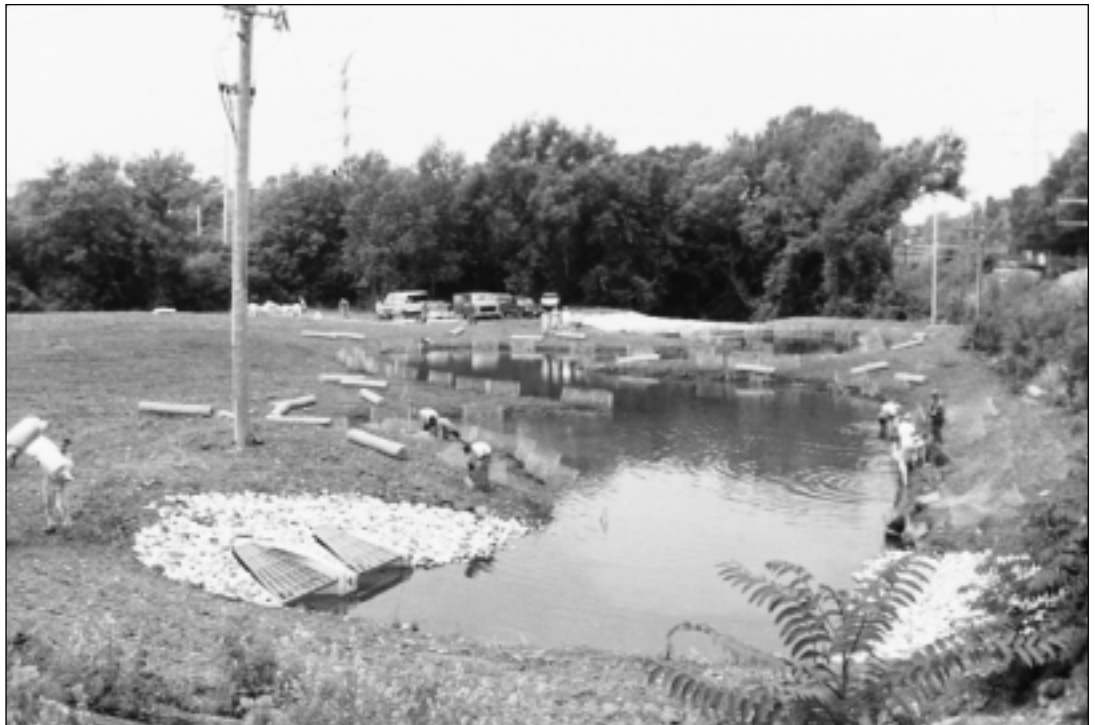
Kilgoblin Wetland after construction. Crews seed the banks, install protective cages around plantings, and prepare to roll out erosion control blankets. Grates cover the two culvert outfalls in the lower left. Courtesy of Village of Barrington Department of Public Works.
