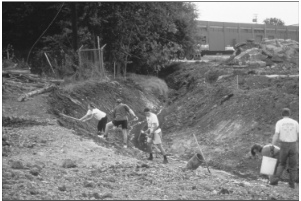
Volunteers working on the banks of the new Codornices Creek channel shortly after excavation. Courtesy of Wolfe Mason Associates.
